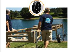
Roll-in is by far the easiest installation. Gradual sloping shorelines with minor obstructions and the lightweight aluminum construction on wheels allows the installer to simply roll the dock in the water. To simplify the installation of the free standing, pile, or pipe supports we have developed a unique float kit. The float kit attaches to the dock frame allowing the installer to float the section into place until the support system is installed.
