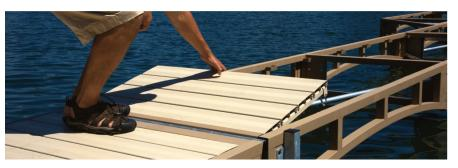
Once the frame sections are positioned, it's time to add the deck. The lightweight, easy-to-handle 2'x4' drop-in deck sections lock into place with spring snaps, no tools needed.
